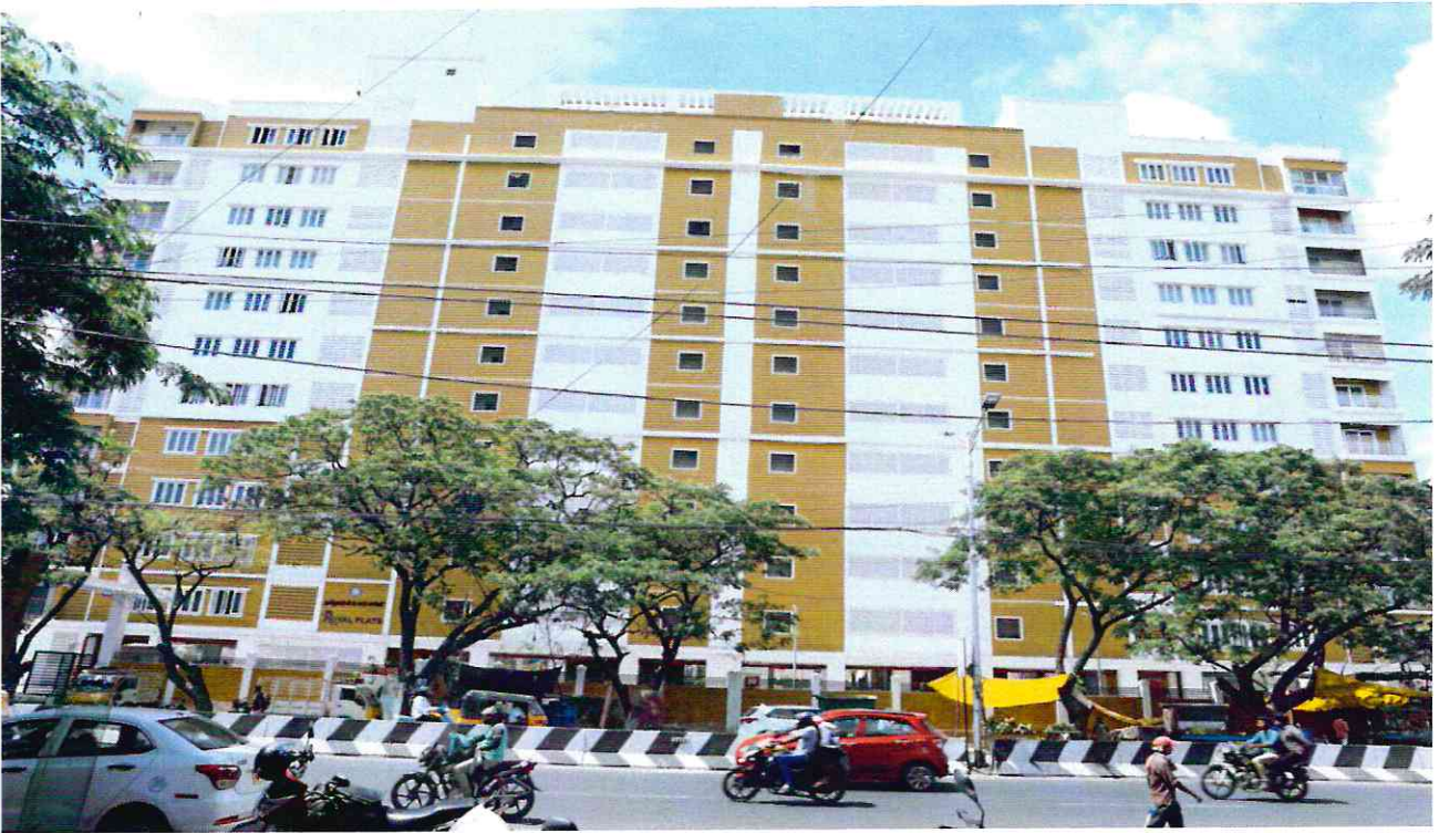
Construction of 44 HIG (Stilt+11 floors) flats at SI No: 195 pt & etc., in Anna Nagar Western Extension (Phase II)
