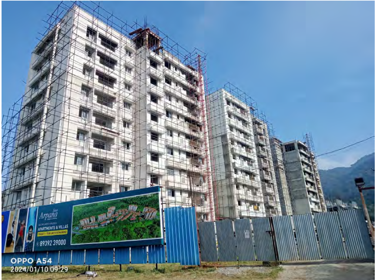
BLOCK D&E TOWER – 1 (Tower K) View -1
