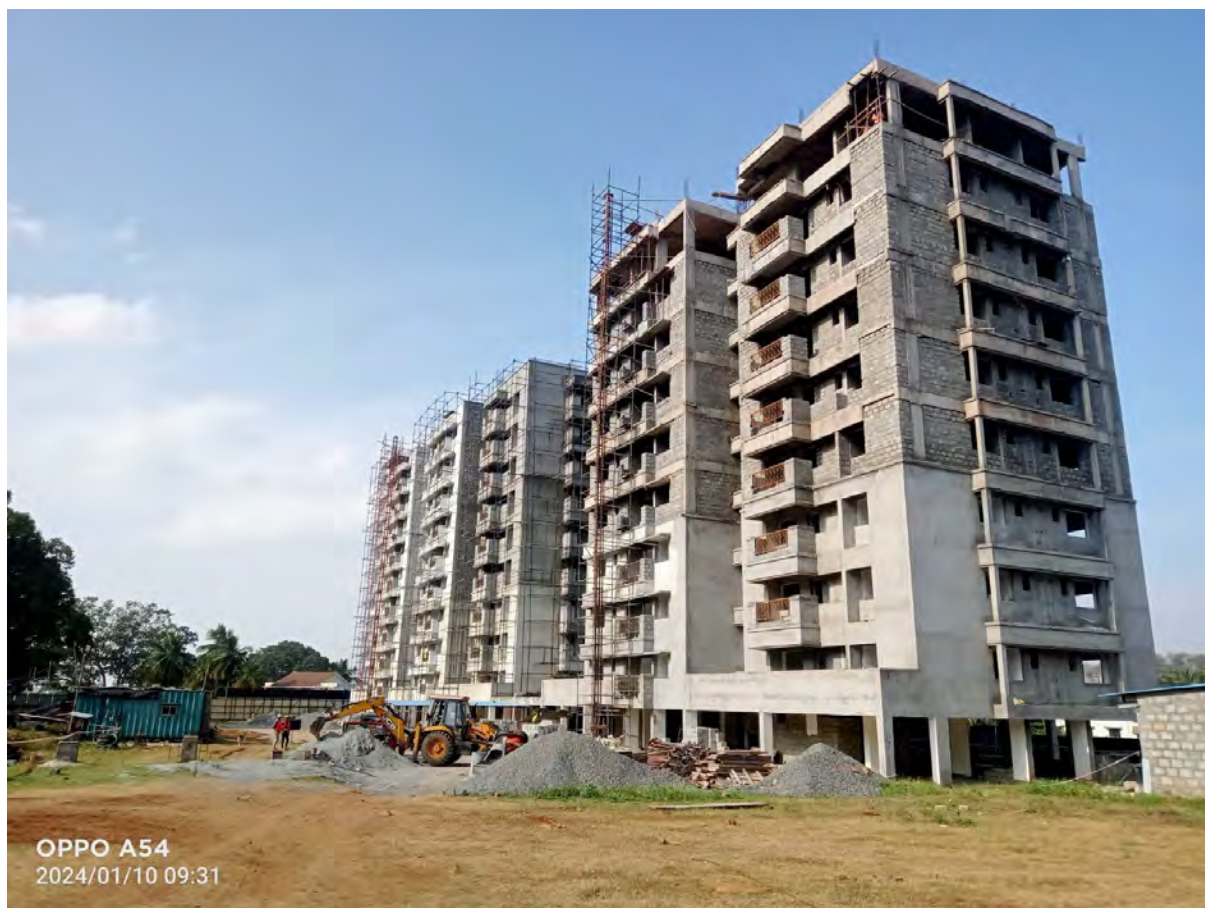
BLOCK D&E TOWER – 1 (Tower K) View -2
