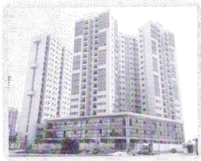
PHASE 1 – JADE, EMERALD & PEARL TOWERS
