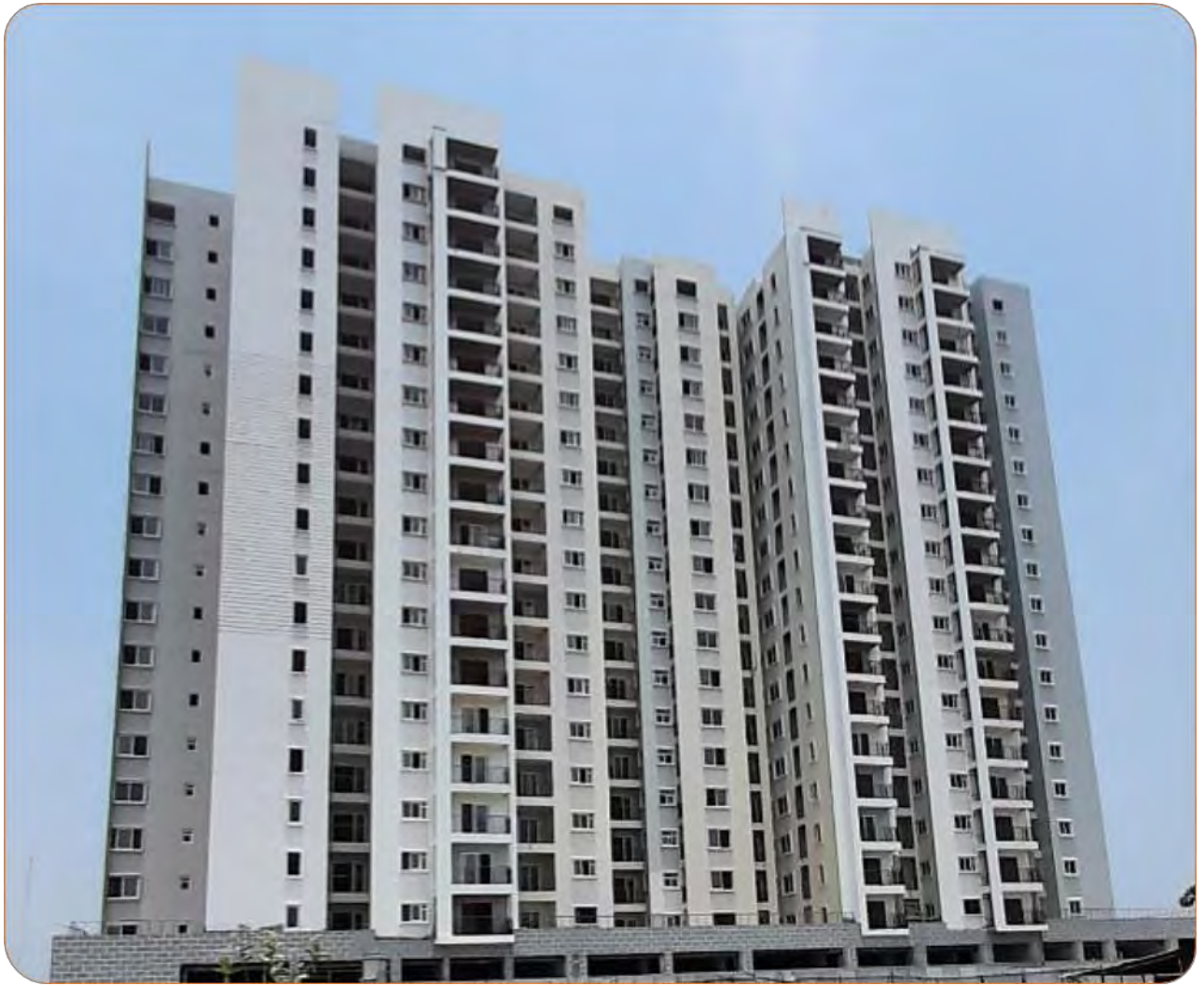
C7 Tower South Side View
