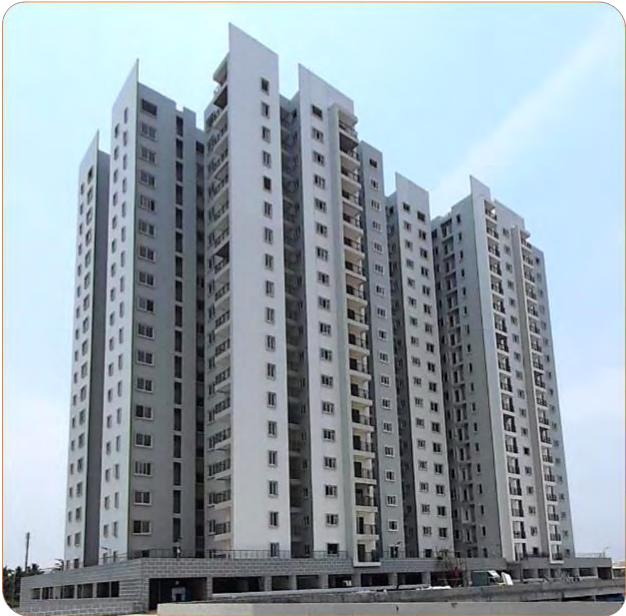
C7 Tower North East Side View
